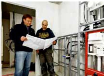
Instruction on site
