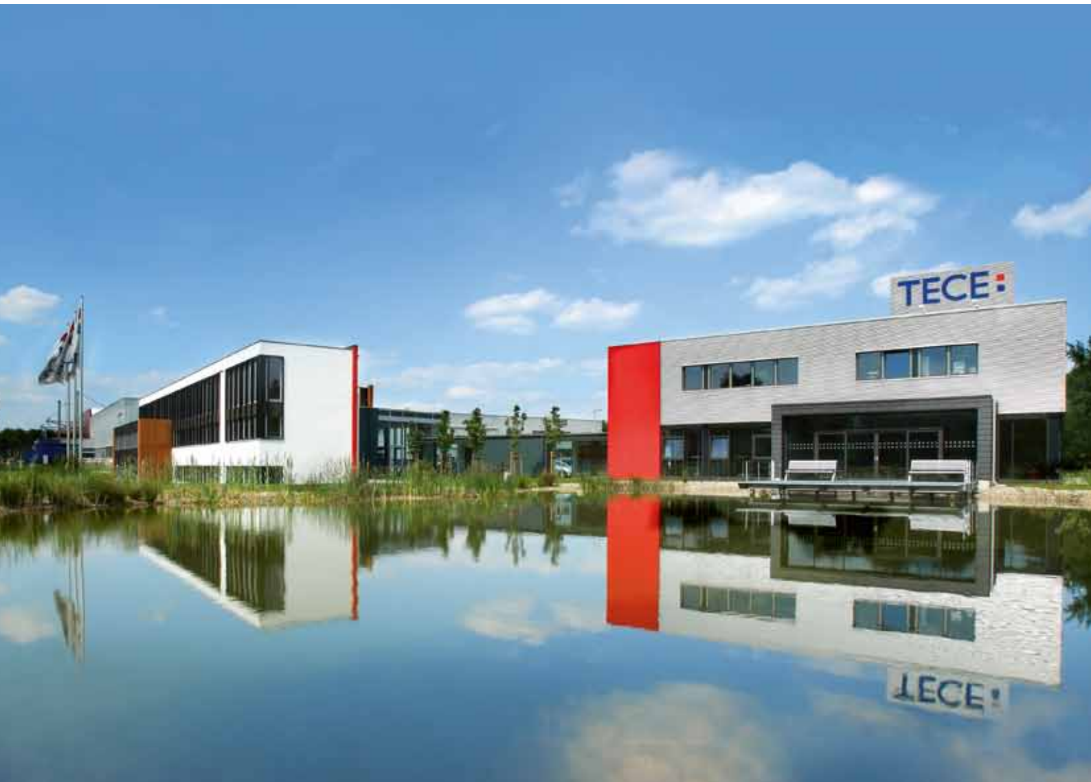
TECE head office with training centre, Emsdetten
