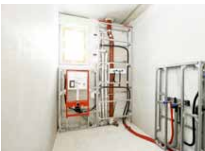
TECEsystem after assembly
